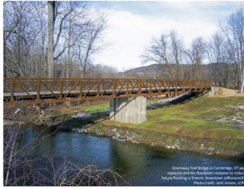
Greenway Trail Bridge in Cambridge, VT
